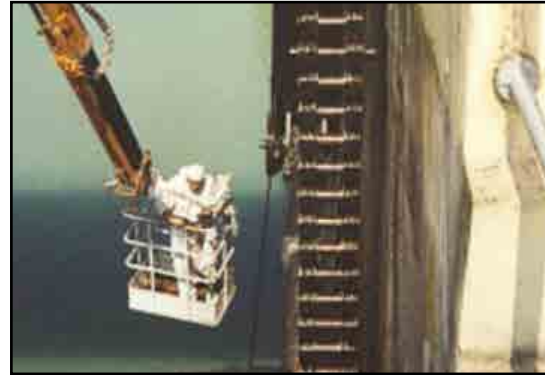
Three products cleaned and restored the chain.
